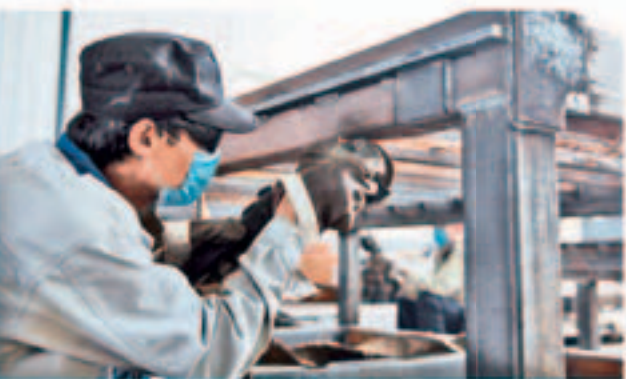
02/ 分段式焊接 Segmented welding
