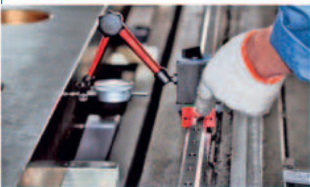
05/ 导轨安装 Rail installation
